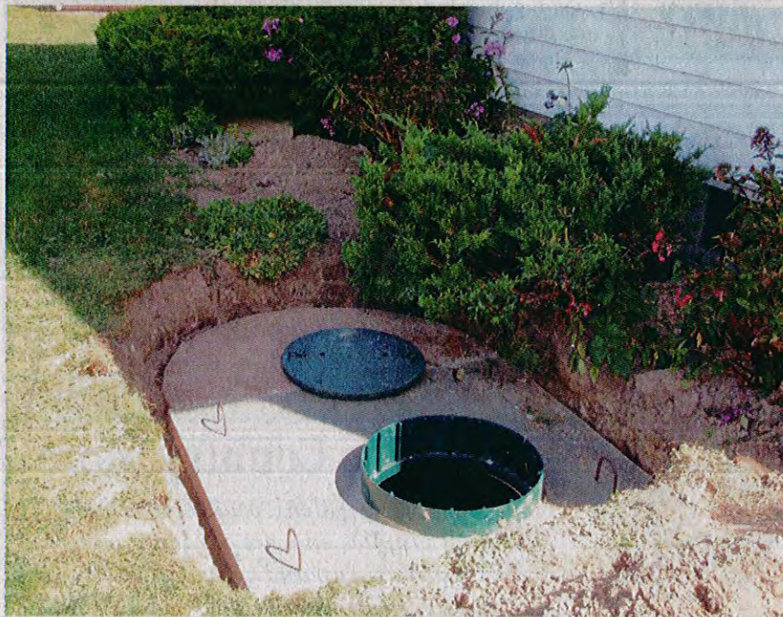
The Lake Huron shoreline, seen from the Point Clark lighthouse, (top) shows the close proximity of cottages and homes, and their septic systems, to the lake. Directly above, a new double chamber septic tank has risers to make it easy to access the tank for pumping and annual cleaning of the filter.
