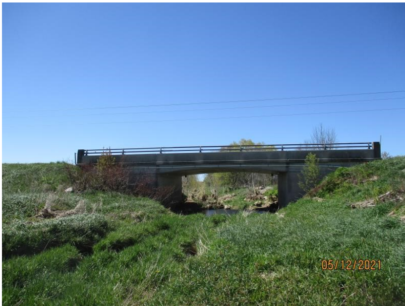
Structure H1 – Concession 2
