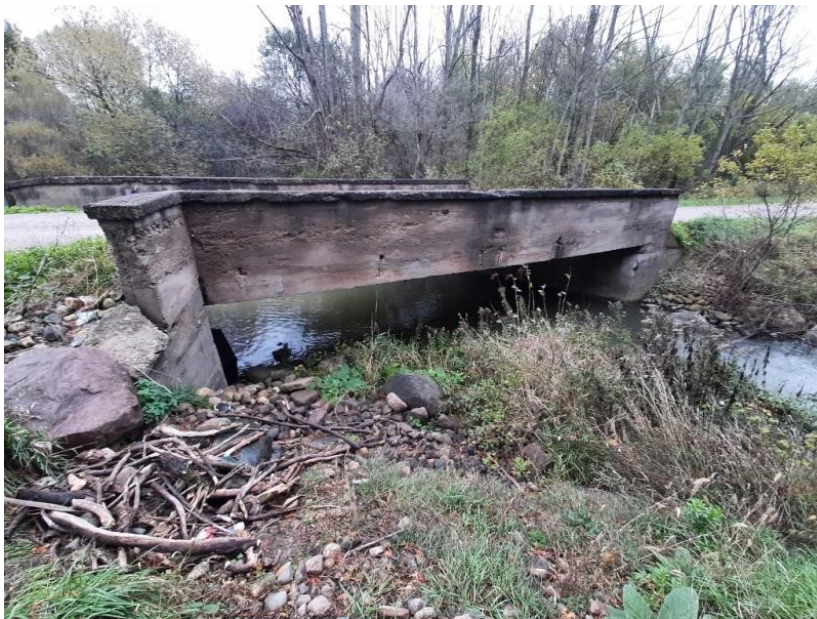
Structure H28 – Sideroad 20
