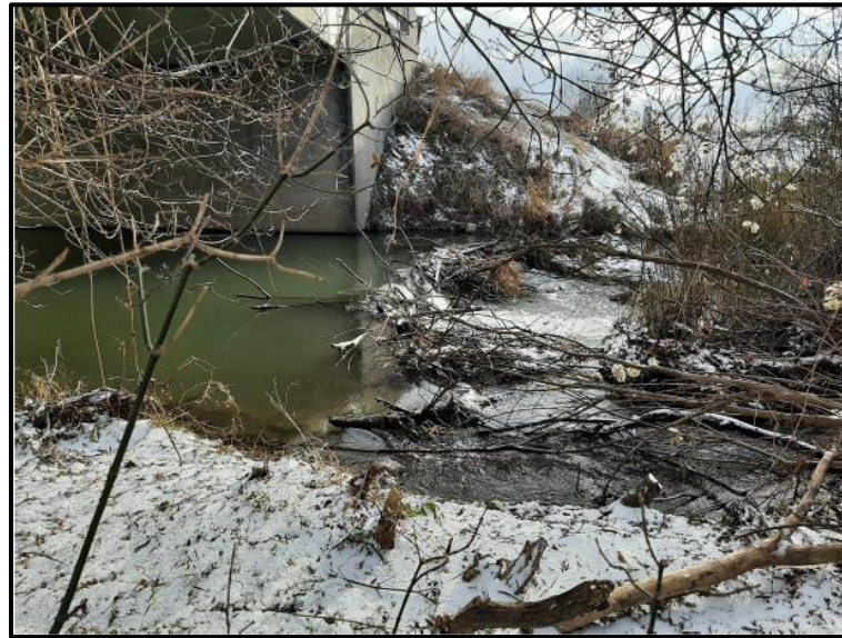
H27 Concession 6 Bridge (BCI =74-Good)
