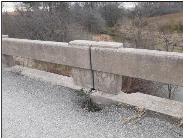
H29 Concession 10 Bridge (BCI = 72- Good)
