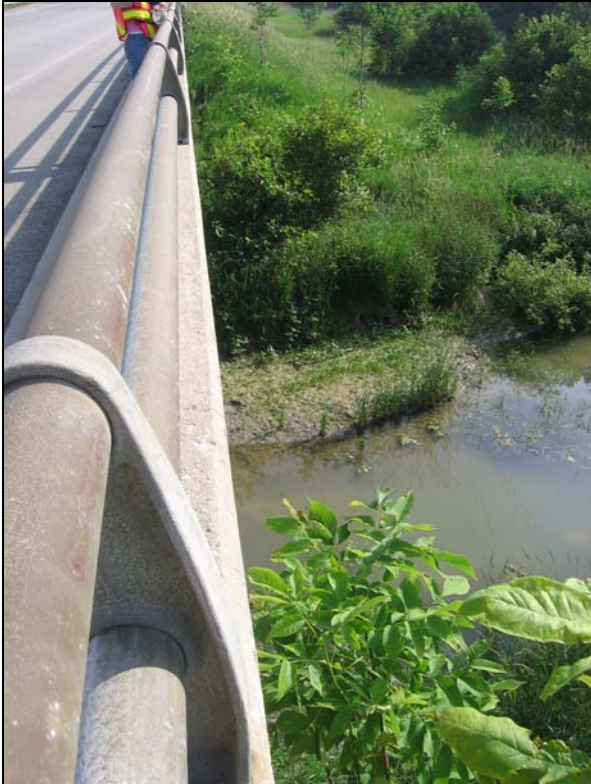
PR 4-Looking across EAST side of bridge
