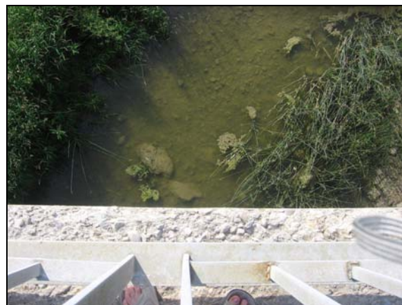
PR 3-Looking down over bridge on EAST side
