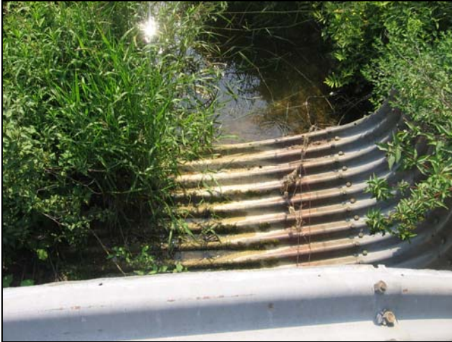
PR 12 –Facing EAST over CSP
