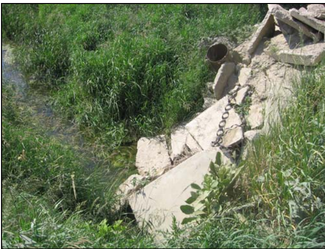
PR 17 – Facing EAST over Concrete Culvert
