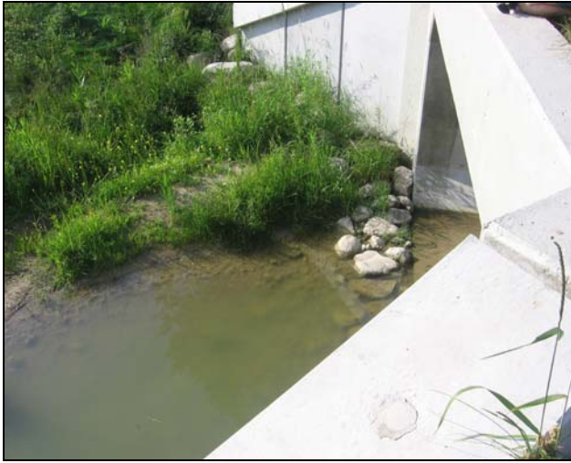
PR 27-Looking across EAST side of culvert
