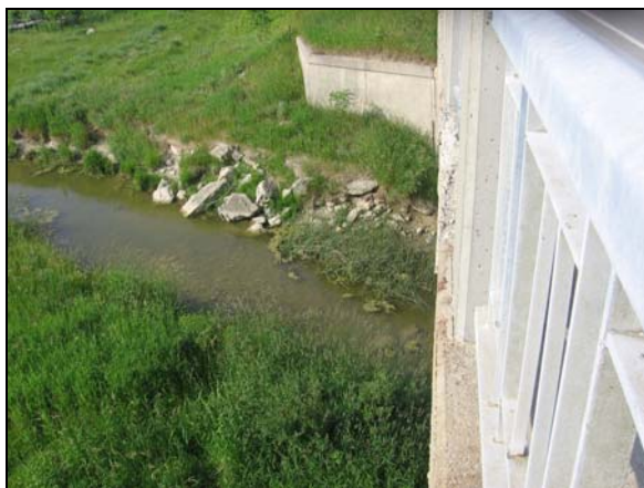
PR 3-Looking across EAST side of bridge
