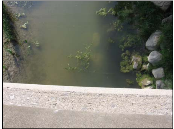
PR 4- Looking down over bridge on EAST side
